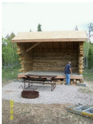
Newly rebuilt warming hut
